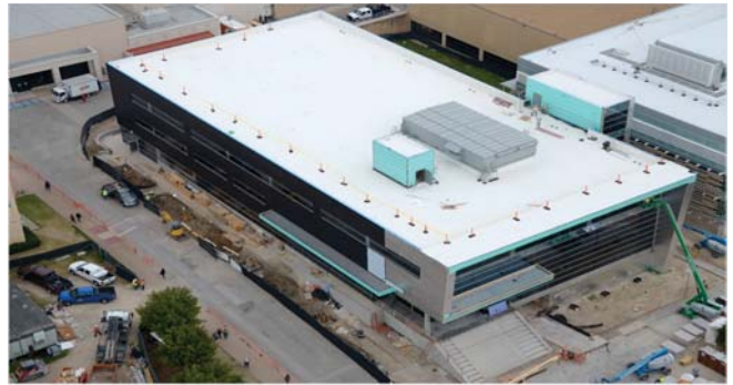
J E Dunn Construction
