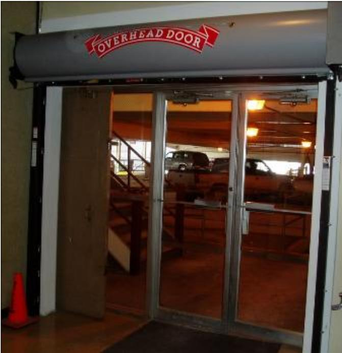
The doors are designed to separate fire areas within a building or protect the means of egress in the event of a fire, thereby limiting its spread.
